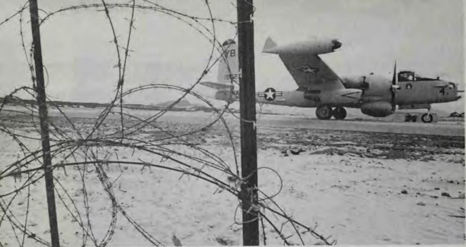
An SP-2H Neptune taxis behind barbed wire at the airstrip at Cam Rahn Bay. Note that the starboard wingtip of this VP-4 aircraft has the standard fixed fuel tank with searchlight mounted in the forward section. The bulge visible under the fuselage is for AN/APS-20 surface search radar. (U.S. Navy, William M. Powers)
