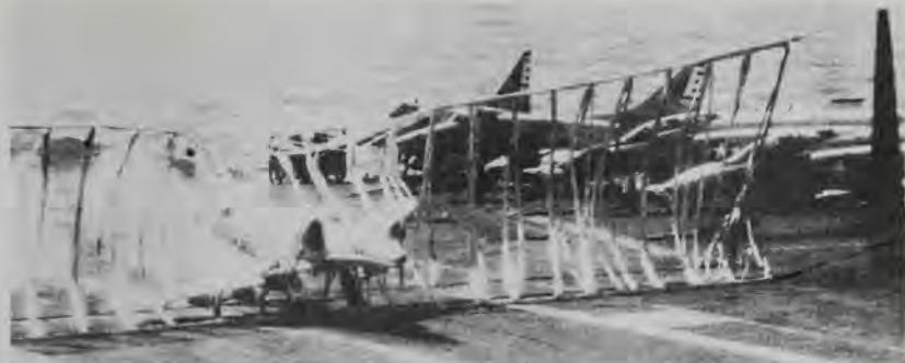
A damaged A-4 Skyhawk slams into the nylon barrier stretched across the angled deck of the *Coral Sea*. The barriers were rigged only when a plane landed with damage and would be unable, if it missed an arresting wire, to take off and come around for another landing attempt. (U.S. Navy)
