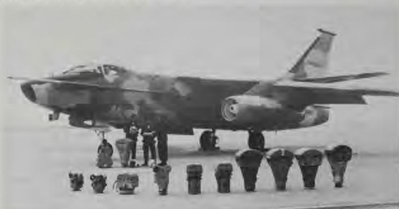
A camouflaged RA-3B Skywarrior and its twelve cameras rest on the runway at Guam before a flight to Southeast Asia. Guam was a staging point for the Navy and the operating base for Air Force B-52s, with the latter also operating out of Thailand. Thirty "Whales" were delivered to the Navy in the RA-3B configuration (originally A3D-2P). The twin 20-mm cannon originally fitted in the tail of this aircraft have been replaced by electronic equipment. (U.S. Navy)
