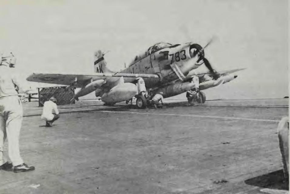
This is an EA-1E electronic warfare variant of the Skyraider from Airborne Early Warning Squadron (VAW) 33, about to be catapulted from the carrier *Intrepid* in the Gulf of Tonkin. The EA-1E (formerly AD-5W) is easily identified by its large cockpit and electronic pods, with the high 700-series number indicating a special-mission aircraft rather than a "straight" attack aircraft. (U.S. Navy, R.A. Lucas)
