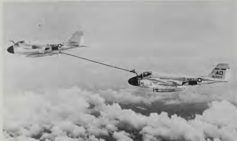
As the venerable "Whales" were phased out of the fleet, the in-flight refueling role was taken over by specifically configured KA-6D Intruders. Here a prototype Intruder tanker refuels an A-6A attack aircraft from VA-42 during flight tests. (Grumman)
