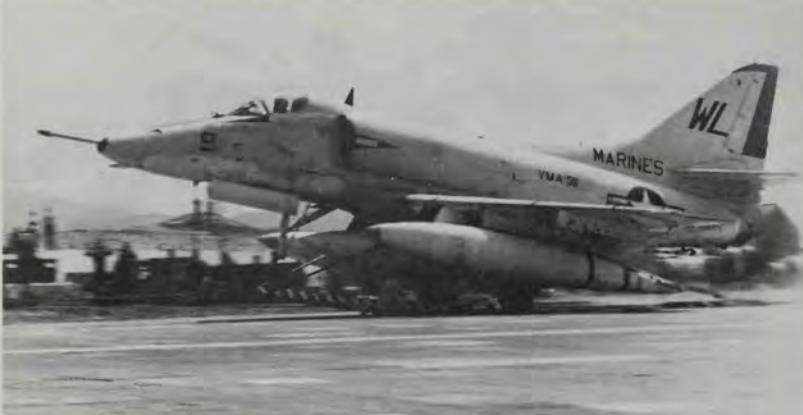
This Marine A-4 Skyhawk is making the first "official" catapult launch from the Marine airfield at Chu Lai on 10 May 1966. During the 1960s the Marines developed catapults, arresting gear, and metal runways for use in forward areas. But most of the massive American complex of airfields built in South Vietnam and Thailand during the 1960s were constructed of concrete. (U.S. Marine Corps)
