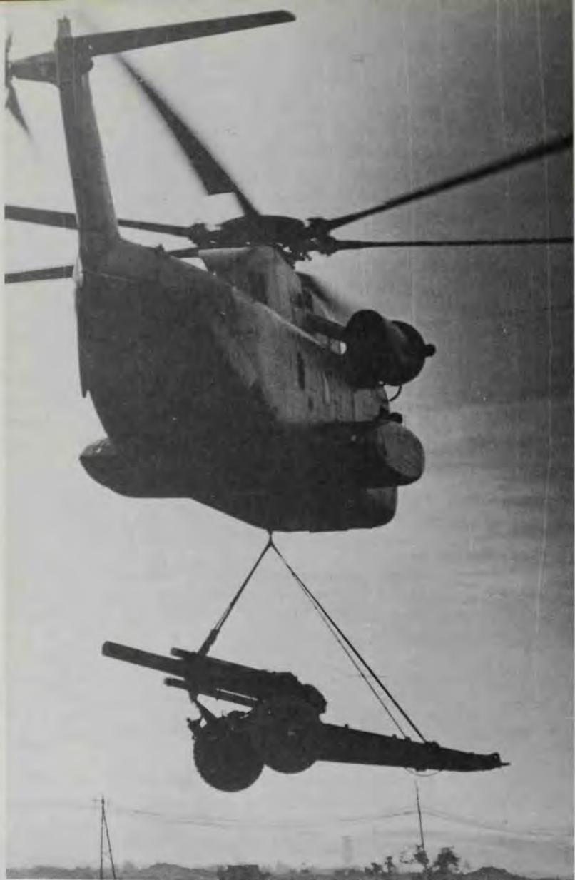
A CH-53A Sea Stallion of Marine Heavy Helicopter Squadron (HMH) 463 lifts a 155-mm howitzer weighing over six tons from the Marine base at Chu Lai to an advanced fire support base. The U.S. Army, Navy, Air Force, and Marine Corps employed several thousand helicopters in the Vietnam War. Note the streamlined lines of the CH-53A when its wheels are retracted and rear loading ramp is closed. (U.S. Marine Corps, Robert Leak)
