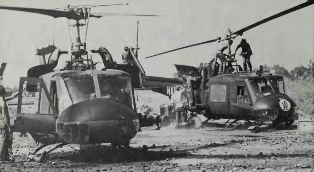
Maintenance personnel work on two UH-1B "Huey" helicopters from HAL-3 "on the beach" in the Mekong Delta area. Helicopters from the "Seawolf" squadron were mainly based on ships and barges in the Delta, but on occasion operated from unimproved landing spots ashore. (U.S. Navy, Dan Dodd)
