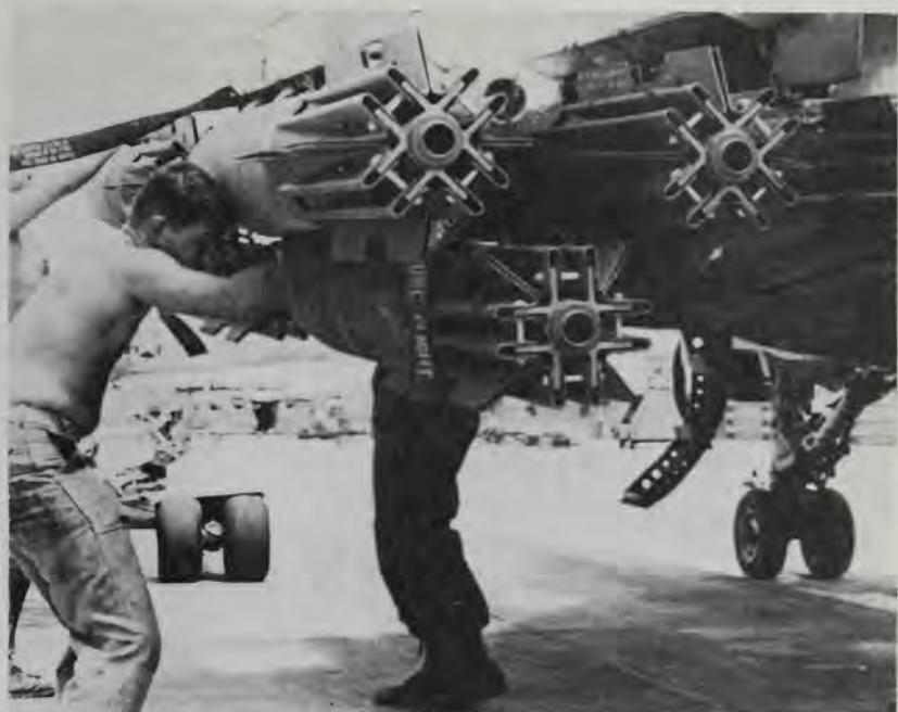
Marine ordnancemen fuse 250-pound Mk-81 bombs aboard attack aircraft at a South Vietnam airfield. The bombs have folding fins that extend after release. (U.S. Marine Corps, C. Stallings)
