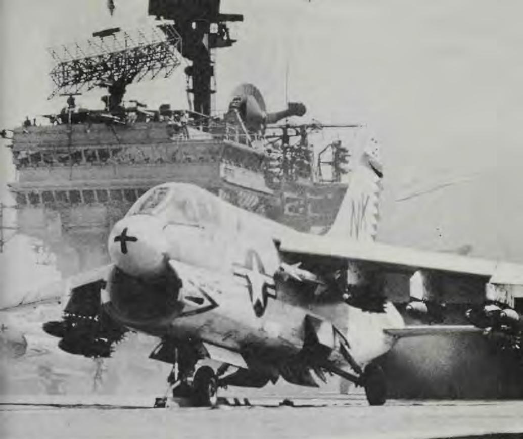
An A-7A Corsair from VA-97 is about to be catapulted from the carrier *Constellation* to strike a target ashore. The black cross on the nose gave early indication to the landing signal officer (LSO) that the plane was an A-7 and not the similar-looking F-8 Crusader. The heavier A-7 required different arresting gear settings; the heavier EA-6B was similarly marked to distinguish it from the A-6. (U.S. Navy)
