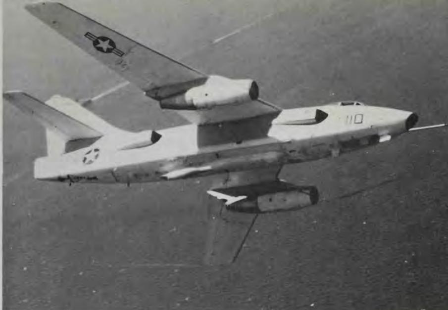
An EKA-3B Skywarrior of Airborne Early Warning Squadron (VAW) 13 from the carrier *Constellation* swings out over the Gulf of Tonkin. Note the electronic "blisters" or fairings along the plane's fuselage. Generally called "Whales," the Skywarriors served extensively in the electronic, tanker, and reconnaissance roles during the war, as well as serving—on a limited basis—as strike aircraft. (U.S. Navy, Paul R. Derby)
