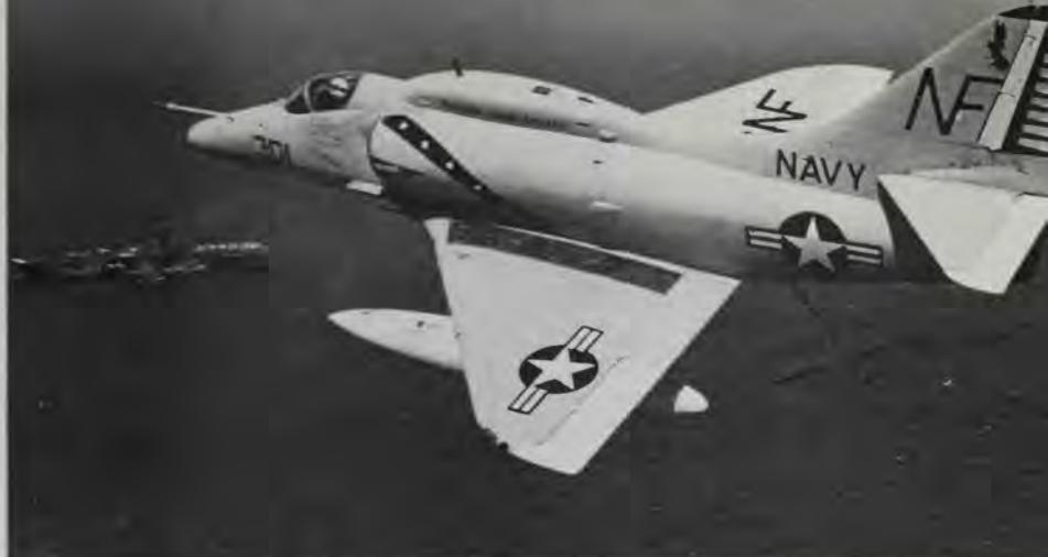
A "humped-back" A-4F Skyhawk from VA-22 on the *Bon Homme Richard* circles over the carrier in preparation for landing as the carrier steams through the Gulf of Tonkin. The A-4 series underwent a continued series of modifications after its original design by Ed Heinemann in the early 1950s as a daylight-only nuclear delivery aircraft. (U.S. Navy, W.E. Bradford)
