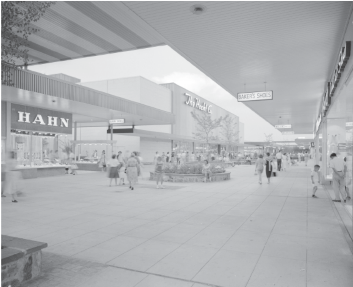
The open-air mall of Prince George Plaza, Hyattsville, Maryland, 1959. Viewed from the inside, the well-appointed, pedestrian-only malls of regional shopping centers belied their reliance on automobiles, creating idealized (and car-free) downtown streetscapes for residents of the booming postwar suburbs. Gottscho-Schleisner Inc., courtesy of Library of Congress Prints and Photographs Division, LC-G613-74127-B.
