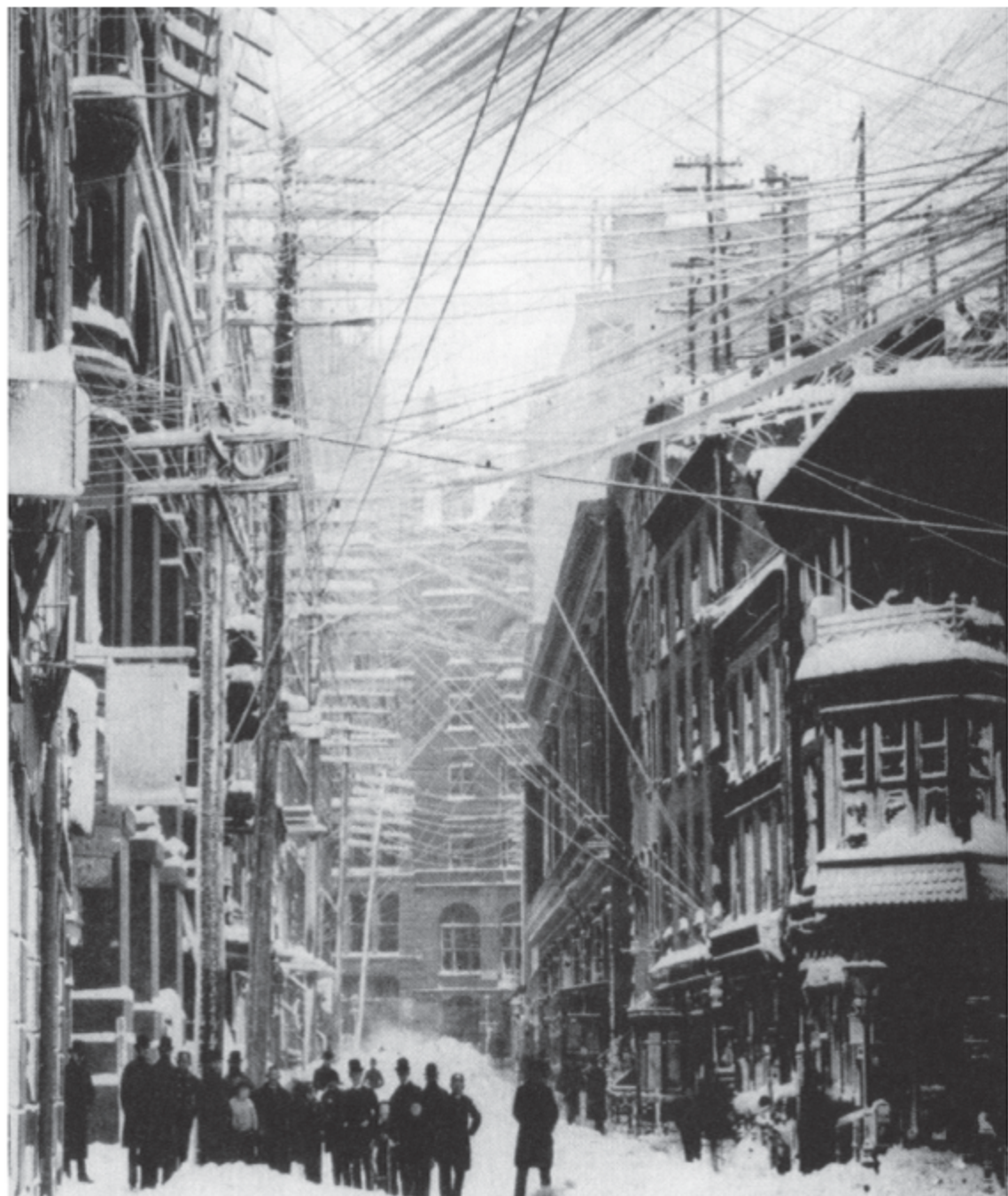
Overhead wires in New York City after the great blizzard of 1888. City dwellers objected both to the unsightliness of overhead wires and to the alarming number of fires and occasional electrocutions that they caused, provoking intense discussions about exactly who had control—and who ought to have control—over decisions that shaped the urban street environment. New York Historical Society.
