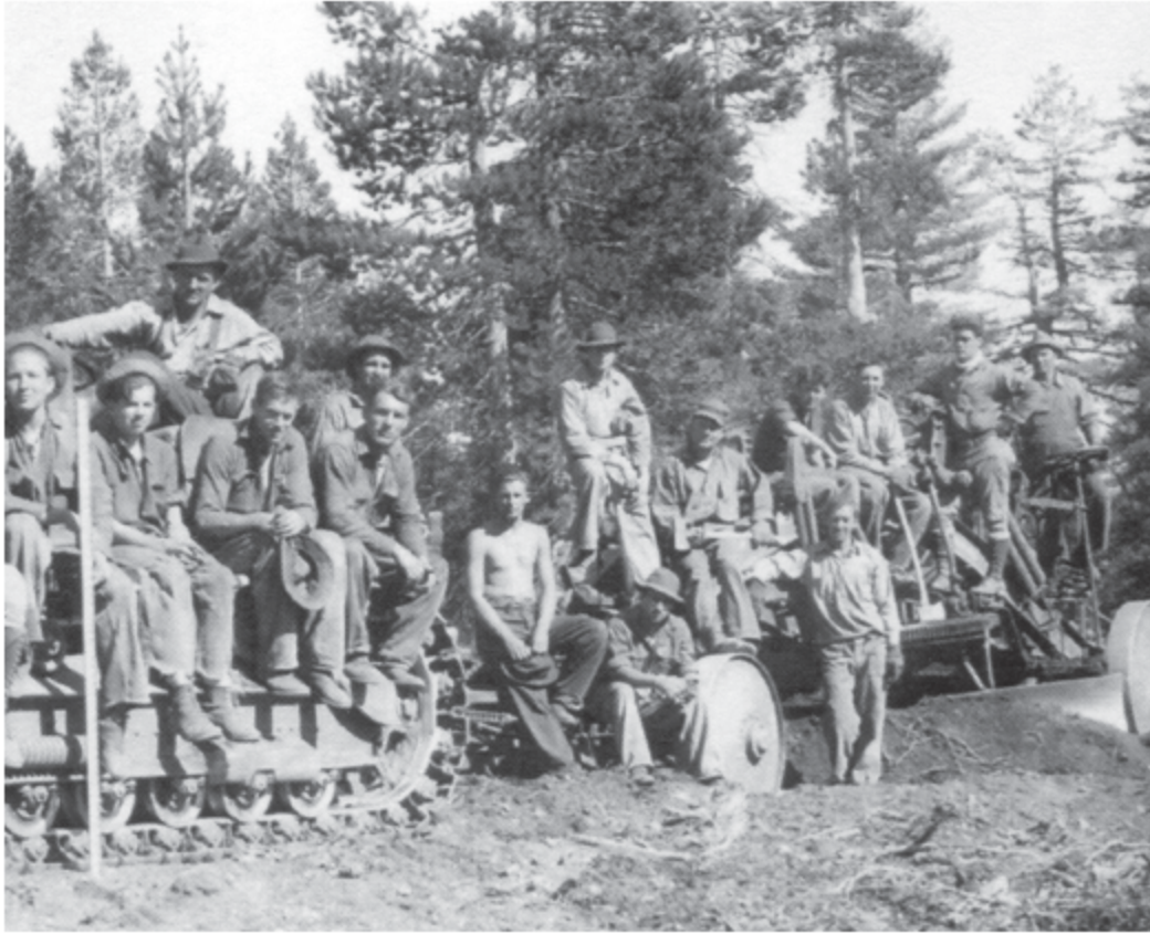
Civilian Conservation Corps road-building crew in the Modoc National Forest, California, 1934. National Archives, NARA 95-G-290289.
