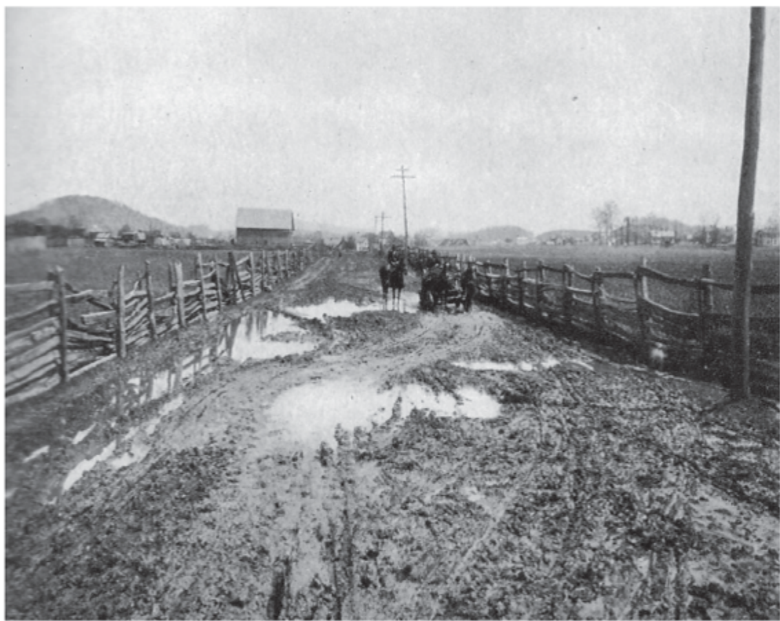
A typical turn-of-the-nineteenth-century rural road. The poor condition of rural highways—characterized by dust in dry weather, mud in wet weather, and rutted, treacherous surfaces year-round—highlighted what reformers saw as the backwardness and isolation of rural farm communities, despite their increasingly sophisticated farm equipment and ready access to urban markets via railroad. From Bureau of Public Roads, Bulletin No. 27 , pl. I, fig. 1.
