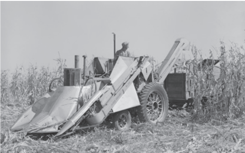
Figure 19.2 Mechanical corn picker, Iowa, 1939. Corn harvesting was a more difficult technical problem than was the case with wheat but was solved from 1939.
