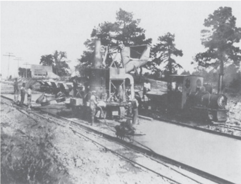
Figure 15.2 Road Construction: North Carolina, 1919. The internal combustion engine wrought a revolution in road construction with the introduction of surface-laying machinery.
