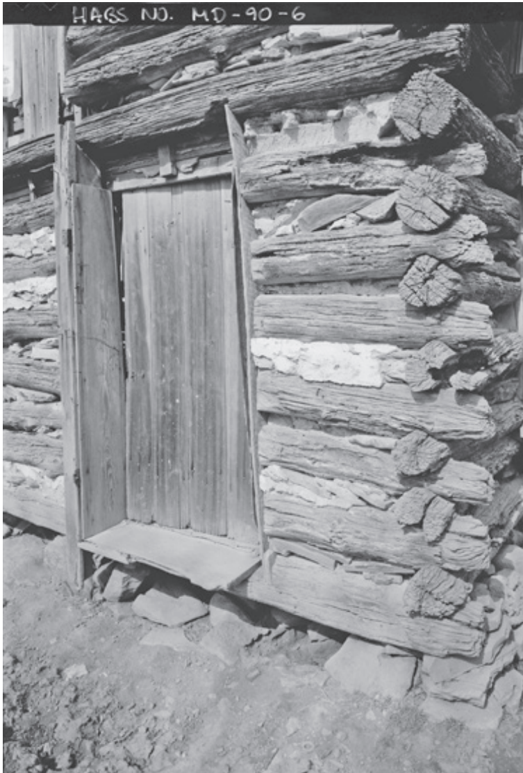
Figure 1.5 An early nineteenth-century log house showing notching and fill between the logs.
