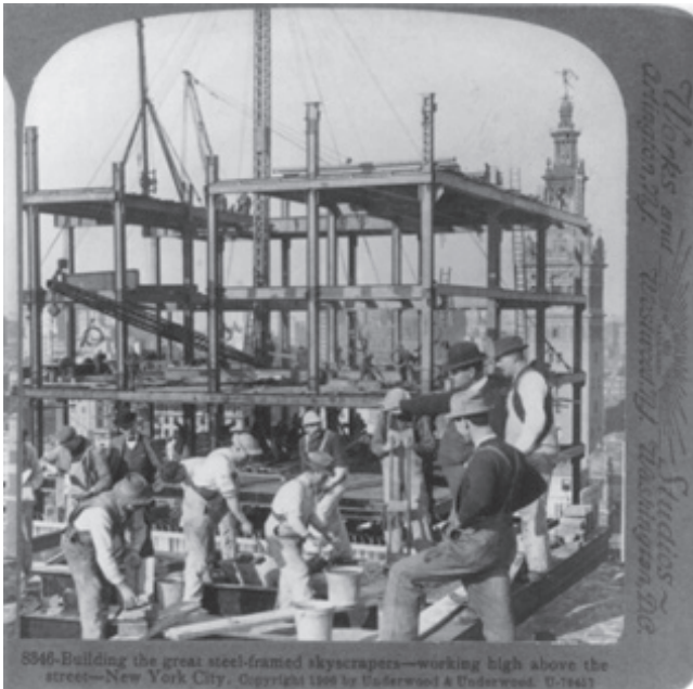
Figure 9.4 Building a steel-framed skyscraper in New York, 1906.
