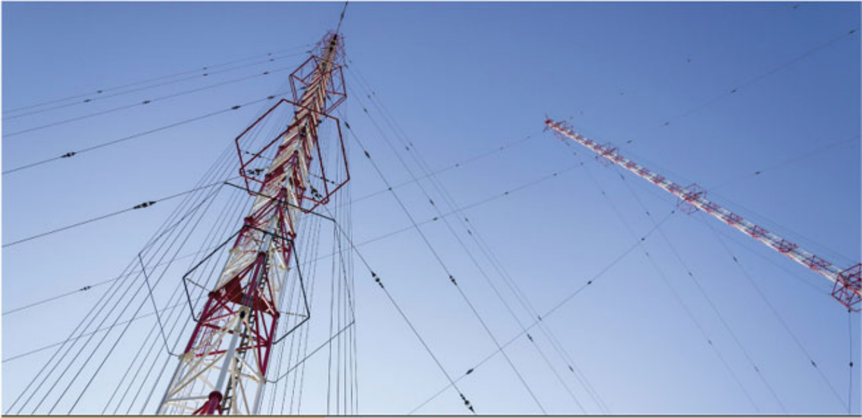
RADIO TOWER WITH GUY-WIRES
