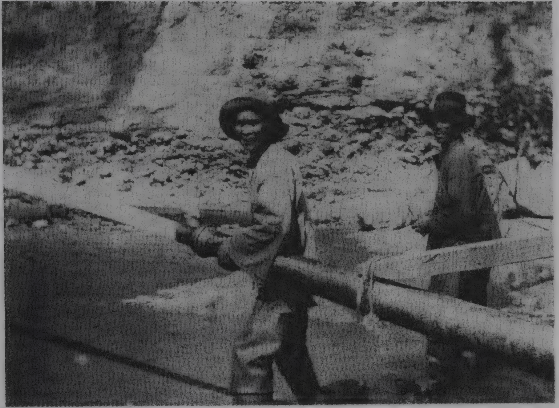
41. Chinese engaged in hydraulic mining in the Rocky Bar region around 1900. Courtesy Idaho State Historical Society, 76-119.2/a.
