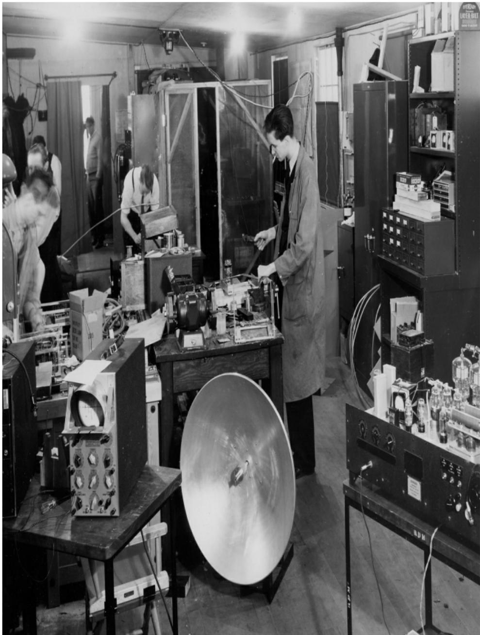
(40) Rad Lab physicists worked around the clock in the Roof Laboratory at MIT to build the first airborne microwave radar system in 1941.
