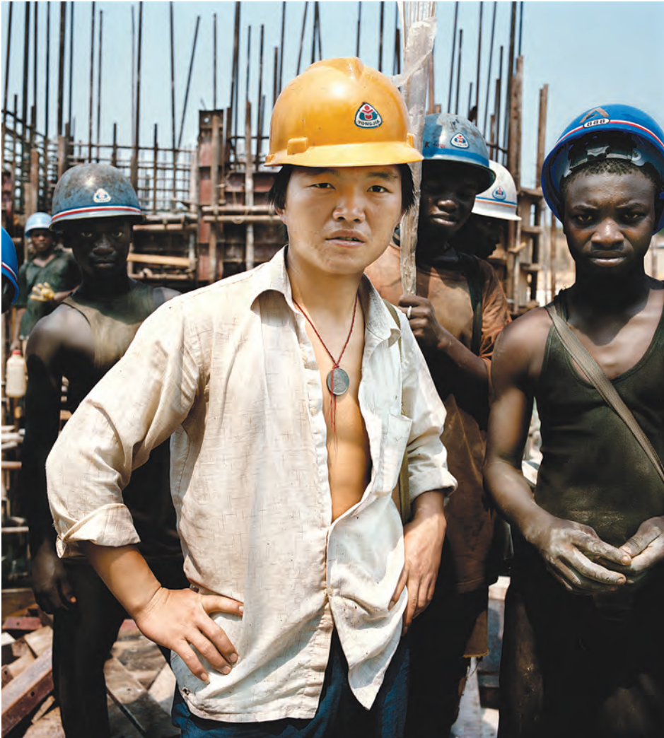
Built not to spill: on the building site of the Imboulou Dam, Congo, 2007
