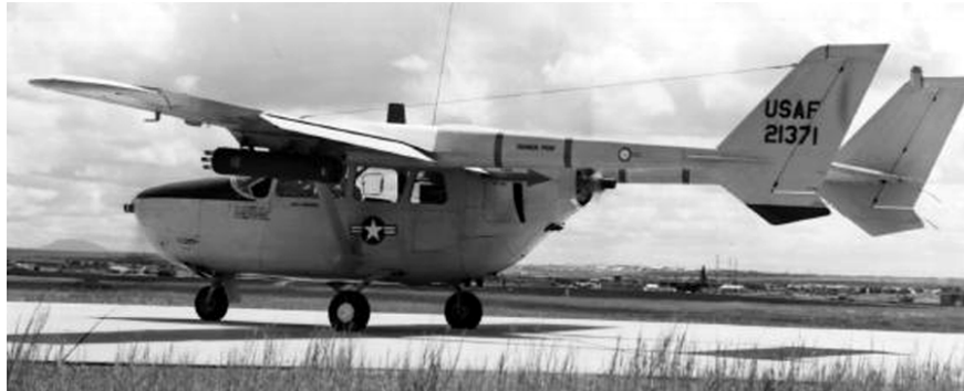
The Cessna O-2 had two engines and hardpoints under the wings.
