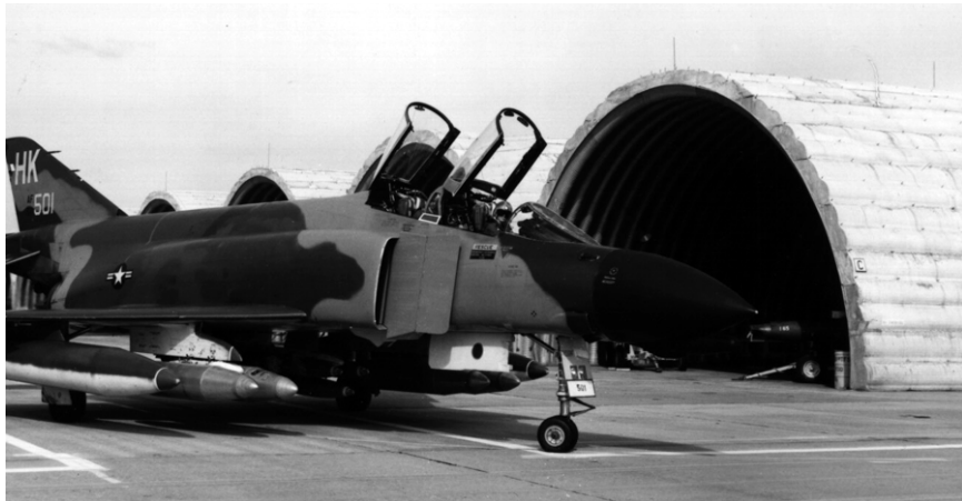
Revetments built before 1968 (top) were open on top and susceptible to rocket attacks from overhead. Shelters built after the 1968 Tet attacks had steel arches on top, covered with eighteen inches of concrete.
